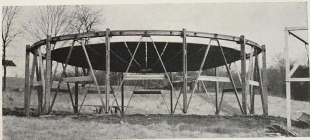
**Cable-hugging** prestressed concrete slabs for suspension roof of Berlin conference hall (AF, Sept. '55) now under construction, use ingenious U-bolt fastening devised by Engineer Fred N. Severud. Slabs for the roof will combat flutter by weight and by serving as transverse ties like strands that tie together long cables of a spider web. Hugh Stubbins, architect; Severud-Elstad-Kruger, engineers.
