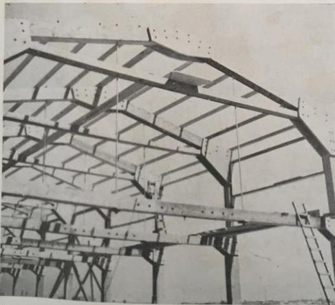
Fig. 1. Rigid frames for this 40x160-ft. building aid in supporting the second floor by means of 1½-in. dia. rod hangers. Gusset plates are of plywood and split ring connectors are used.
