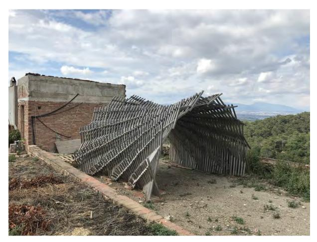
Figure 2.1: The entire shelter was assembled by 6-axis robotic arm, which also formatted each individual wooden beam (Masia Can Valldaura, Barcelona, Spain). Photographed by the author in 2018.
